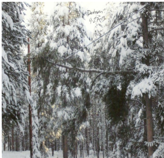
Tree Leaning on Distribution Line in the Big Horn National Forest. Source: Big Horn REA
